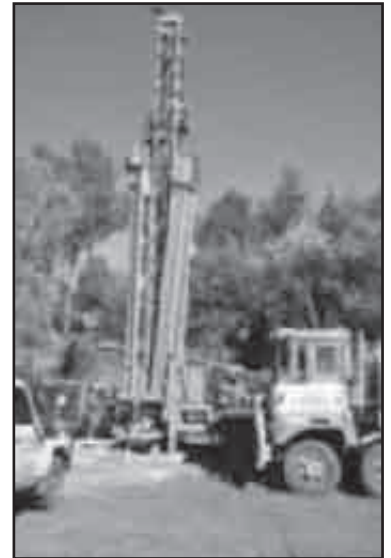
The Frank Walsh drilling team on site at Rostrevor College in 2010
