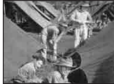
From the 1955 Annual: Erecting tents at Warradale
